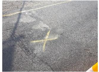
Image 19: Repair to internal asphalt road marked
