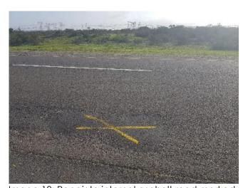
Image 18: Repair to internal asphalt road marked
