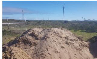
Image 30: Topsoil stockpile
